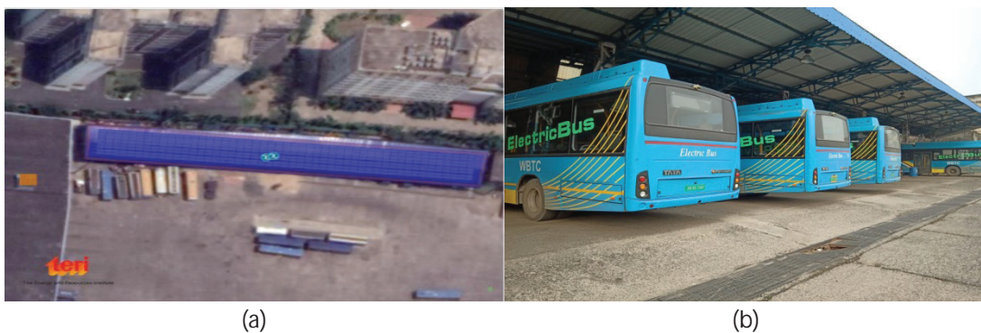
Figure I: (a) GIS estimation of RTPV potential in bus depot (b) Electric buses getting charged in the depot
