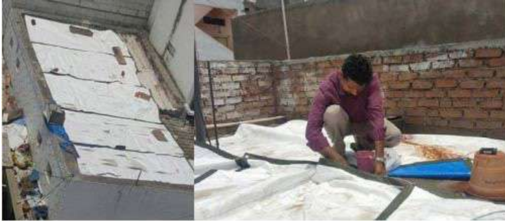
Figure 36: Cool roof pilot installation in Hyderabad [29]
