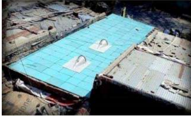
Figure 35: ModRoof installation in Ahmedabad by Mahila Housing SEWA Trust [29]
