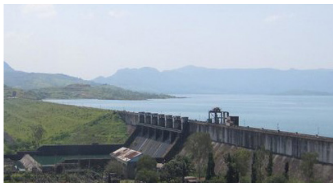
FIGURE 21: Mulshi dam on Mula River near Pune city 53
