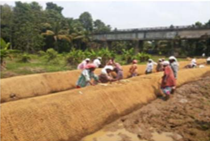
IWMP – IX / 2012-2013, Thodupuzha Block, Idukki – Bund construction with Coir Geo Textiles, Kerala
