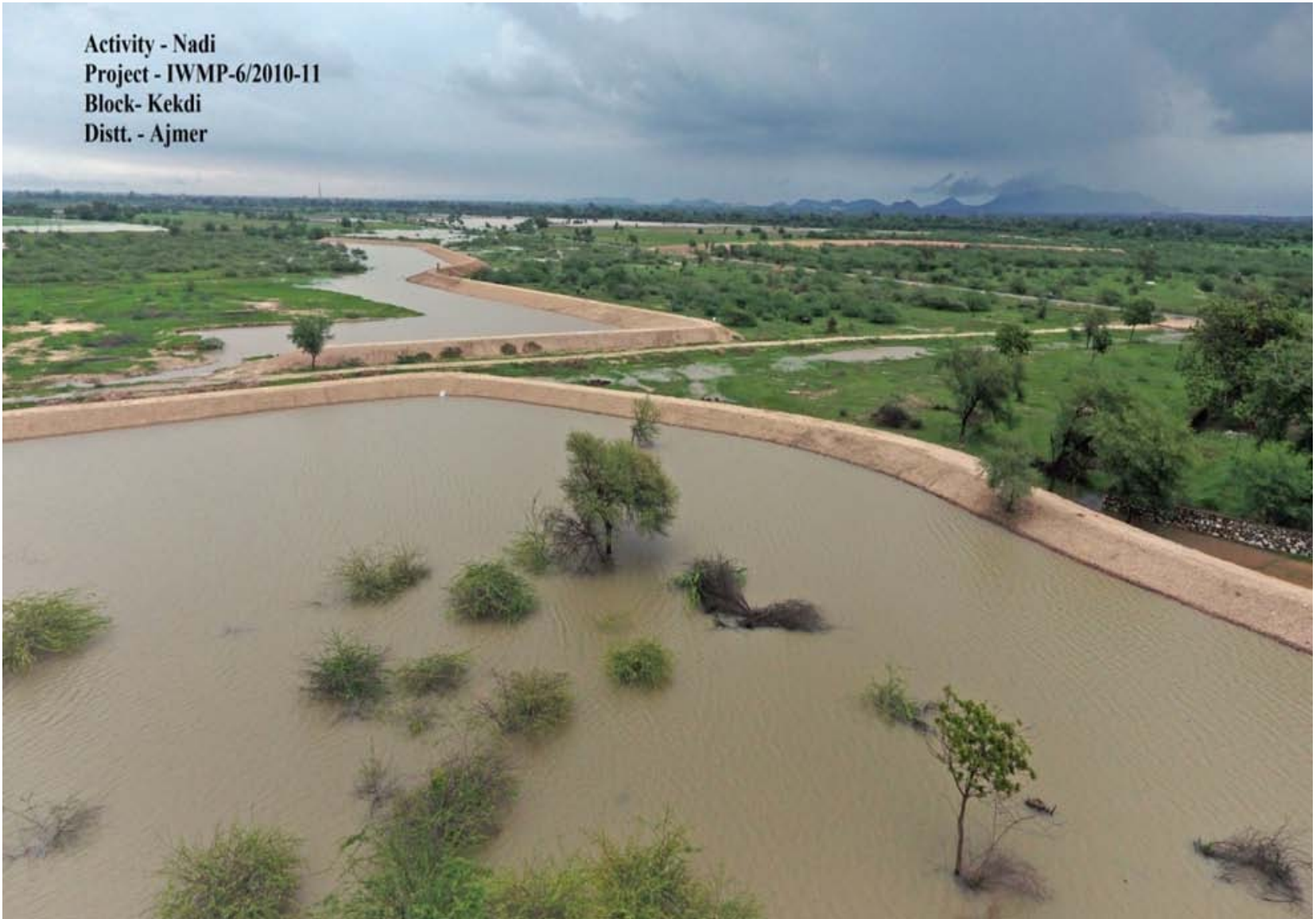
Farm Pond at Ajmer District Rajasthan (IWMP Batch II projects)
