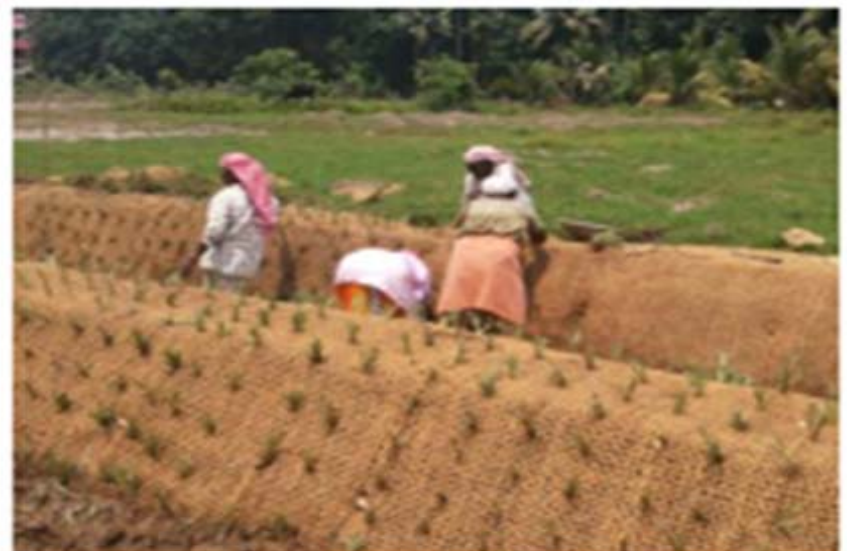
IWMP – IX / 2012-2013, Thodupuzha Block, Idukki – Bund construction with Coir Geo Textiles, Kerala
