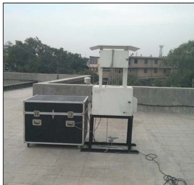
Sampler Installed at the Naraina Site
