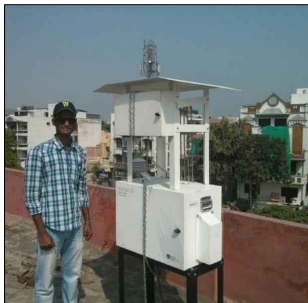
Sampler Installed at the Janak Puri Site
