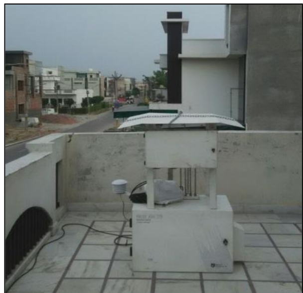
Sampler Installed at Sector 15, Sonipat Site
