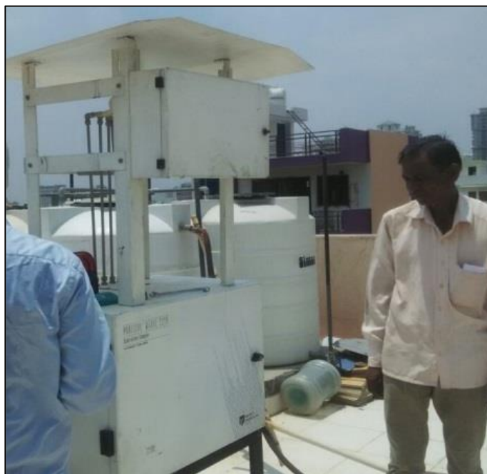
Sampler Installed at HUDA, Sector 43, Gurgaon Site
