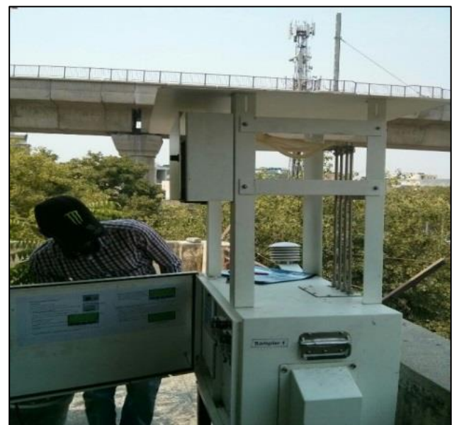
Sampler Installed at the Mayur Vihar Site
