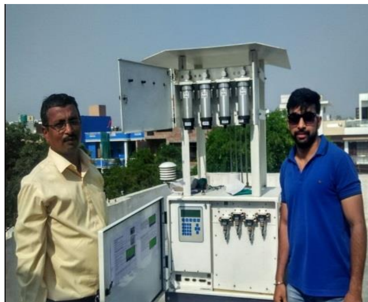
Sampler Installed at HUDA Colony, Panipat
