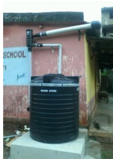
Construction of safe drinking water infrastructure
