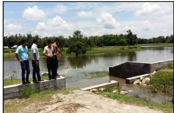
Photos 3: RCC check dam at Bamundanga MWS under Raidak IWMP
