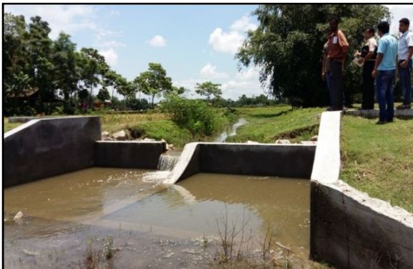
Photos 2: RCC check dam at Bamundanga MWS under Raidak IWMP
