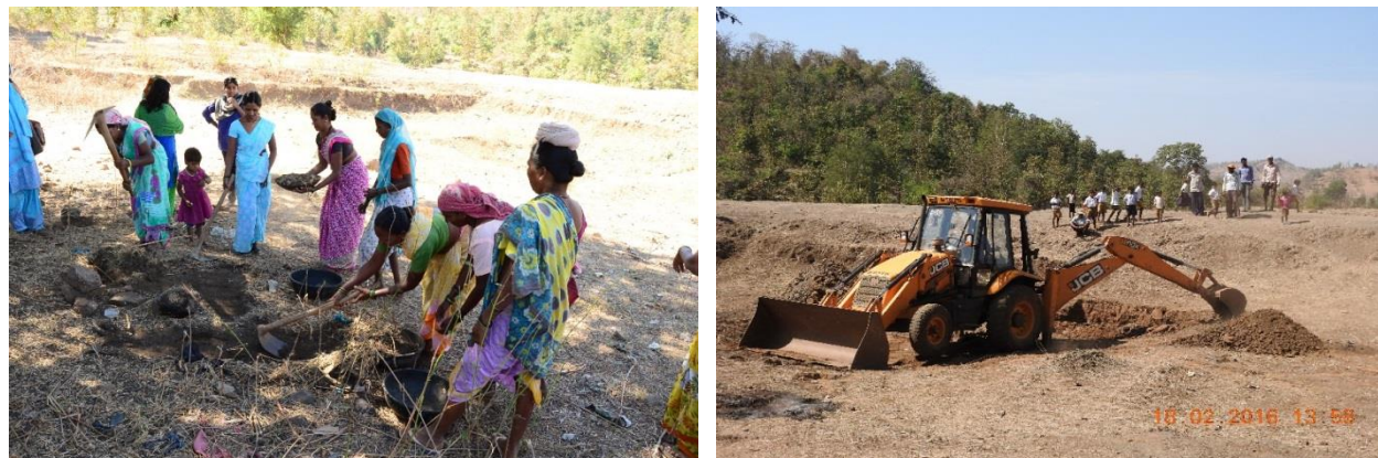
Picture No. 14: De-siltation carried out with community participation and with the help of the mechanical device
