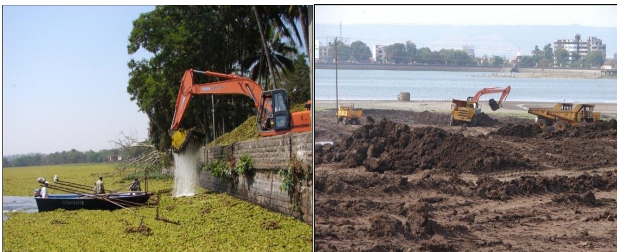
Picture No. 8: De-weeding operation (left) and De-silting (right) at Rankala Lake
