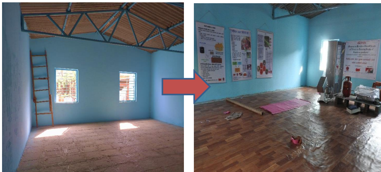
Picture No. 5: The community hall in Vijapur village, before and after its conversion into a food processing unit/ resource centre
