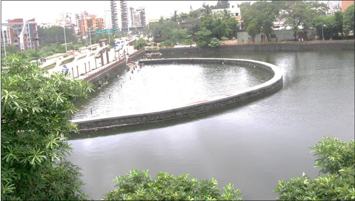
Picture No. 8: Gabion wall partition for restricting idols immersion at Rabale lake
