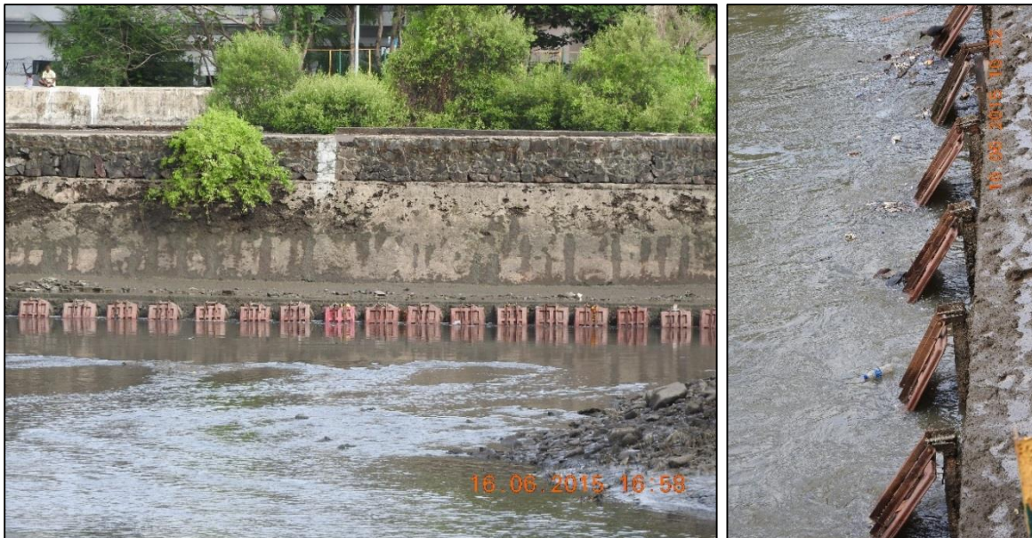
Picture No. 7: Dutch dyke (Holding ponds) with open flap gates at Vashi.
