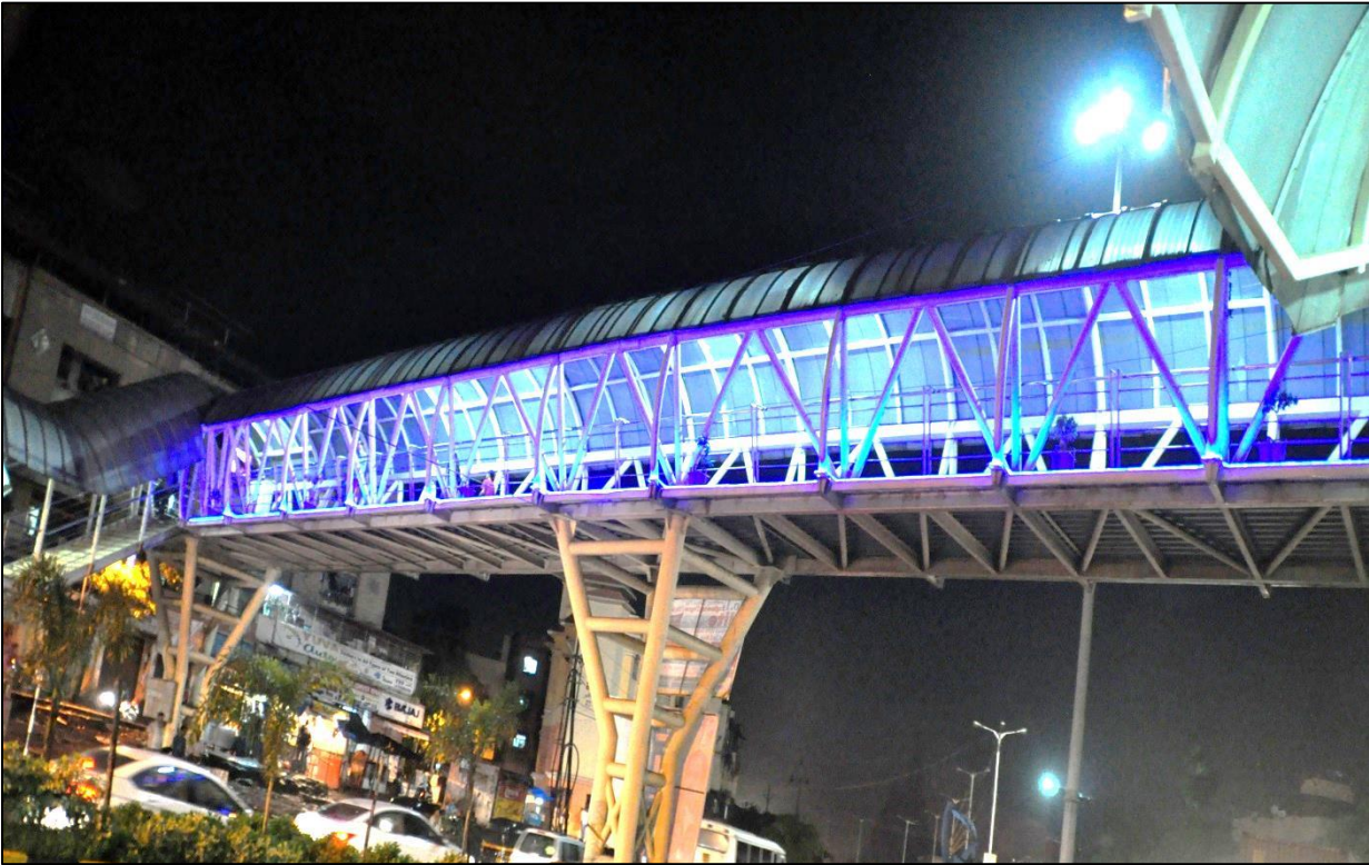
Picture No. 5: Illumination of LED lights installed at Airoli –Diva skywalk
