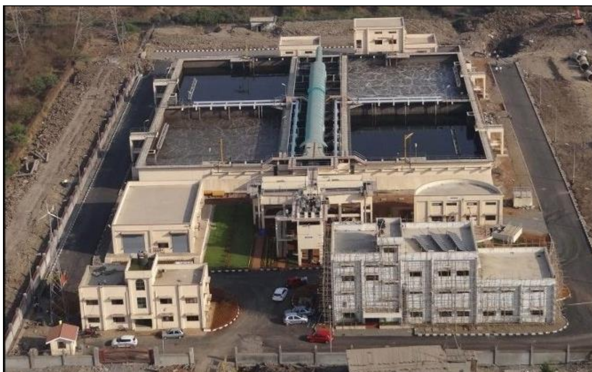
Picture No. 6: Sewage Treatment facility at Sanpada
