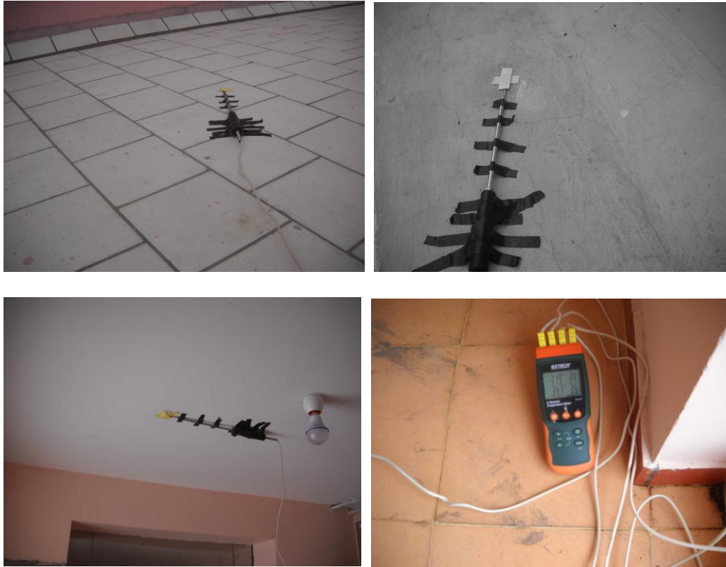
Figure 3 a) Overdeck of Insulla tiled roof; b) Overdeck of conventional roof; c) Underdeck of Insulla tiled roof; d) Datalogger connected to temperature sensors
