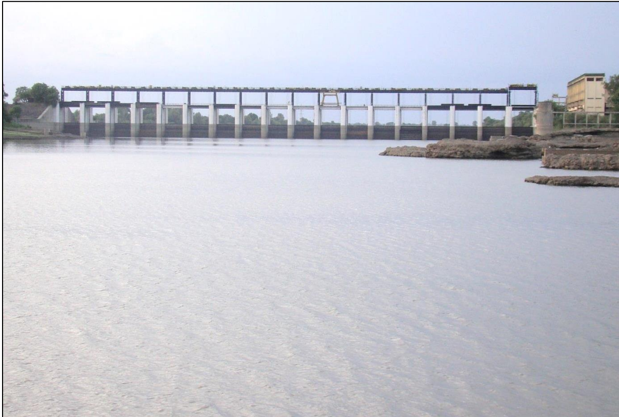
Picture No. 4: Vishnupuri Dam constructed on Godavari River in Nanded
