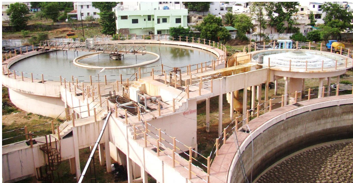
Picture No. 5: View of the Kabra nagar water treatment plant at Nanded
