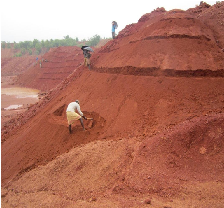
Figure 23 Construction of contour terraces in slope areas of Pakhar plateau
