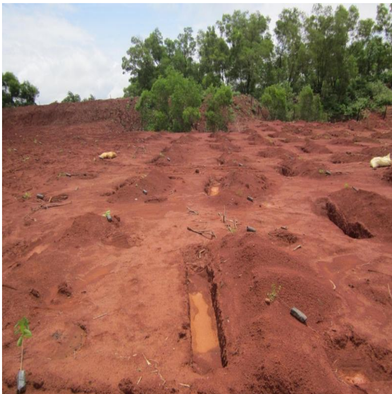
Figure 24 Construction of contour trenches at Bagru plateau
